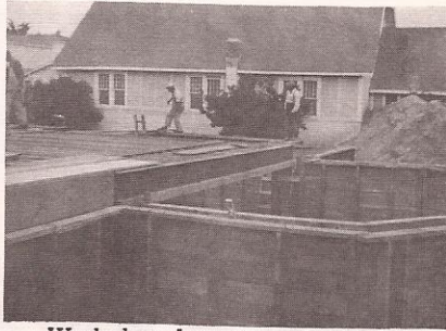
Work has begun — forms for the basement.
