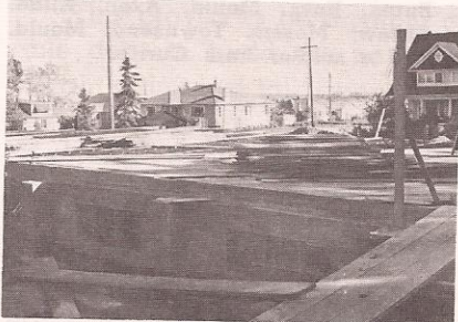
Finally above ground — rough floor laid by volunteers.
